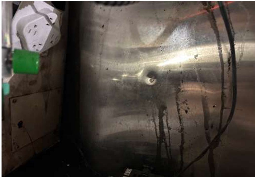
Image 2 - Pilot Hole Close-up
