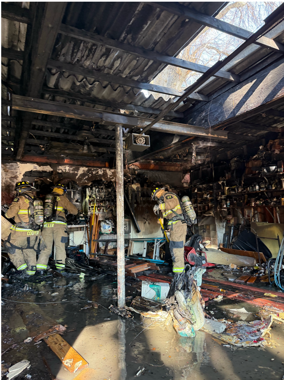
Image 3 - Interior of Garage (Notice the Pooling of the Water/Fuel on the Ground)
