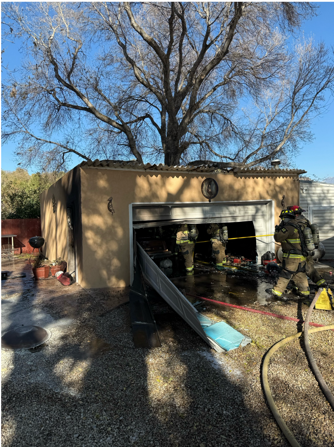
Image 1 - View of the A/B corner of the garage
