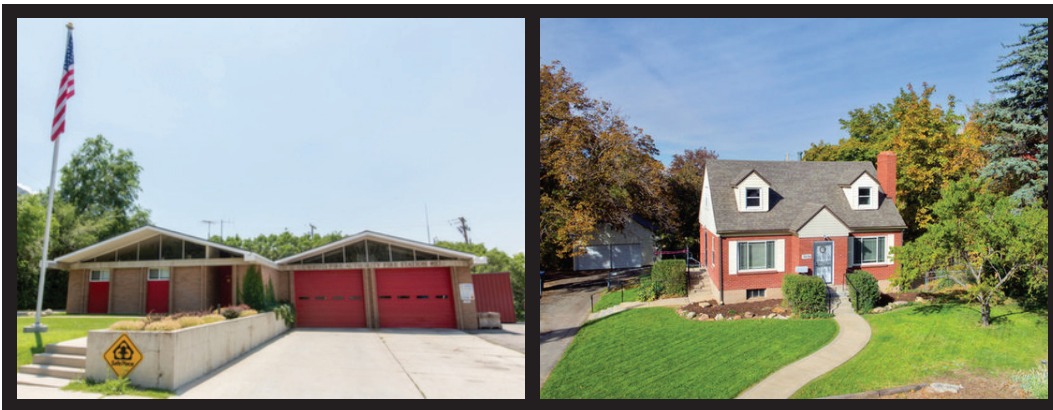
3612 Jupiter Drive - Current site of Station #112 to be rebuilt
