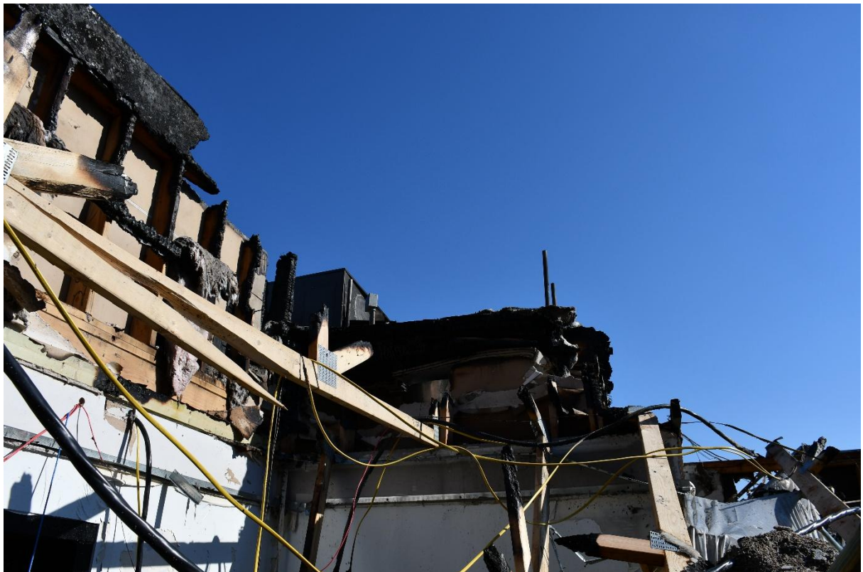
Figure #43 Looking up from the front of Elevators
