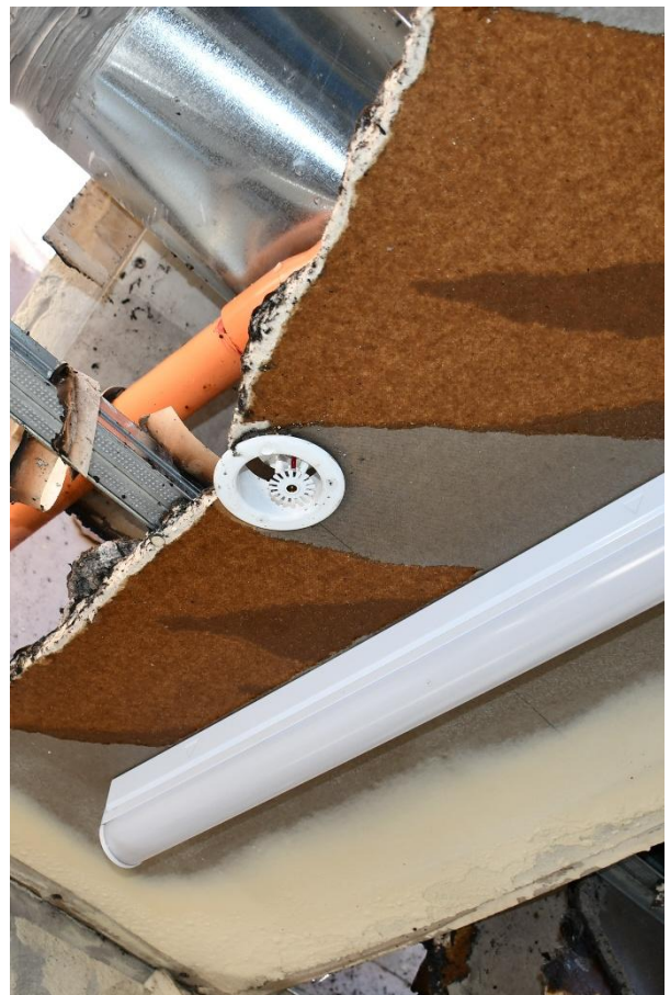
Figure #19-20 Looking at the Fire Sprinkler system
