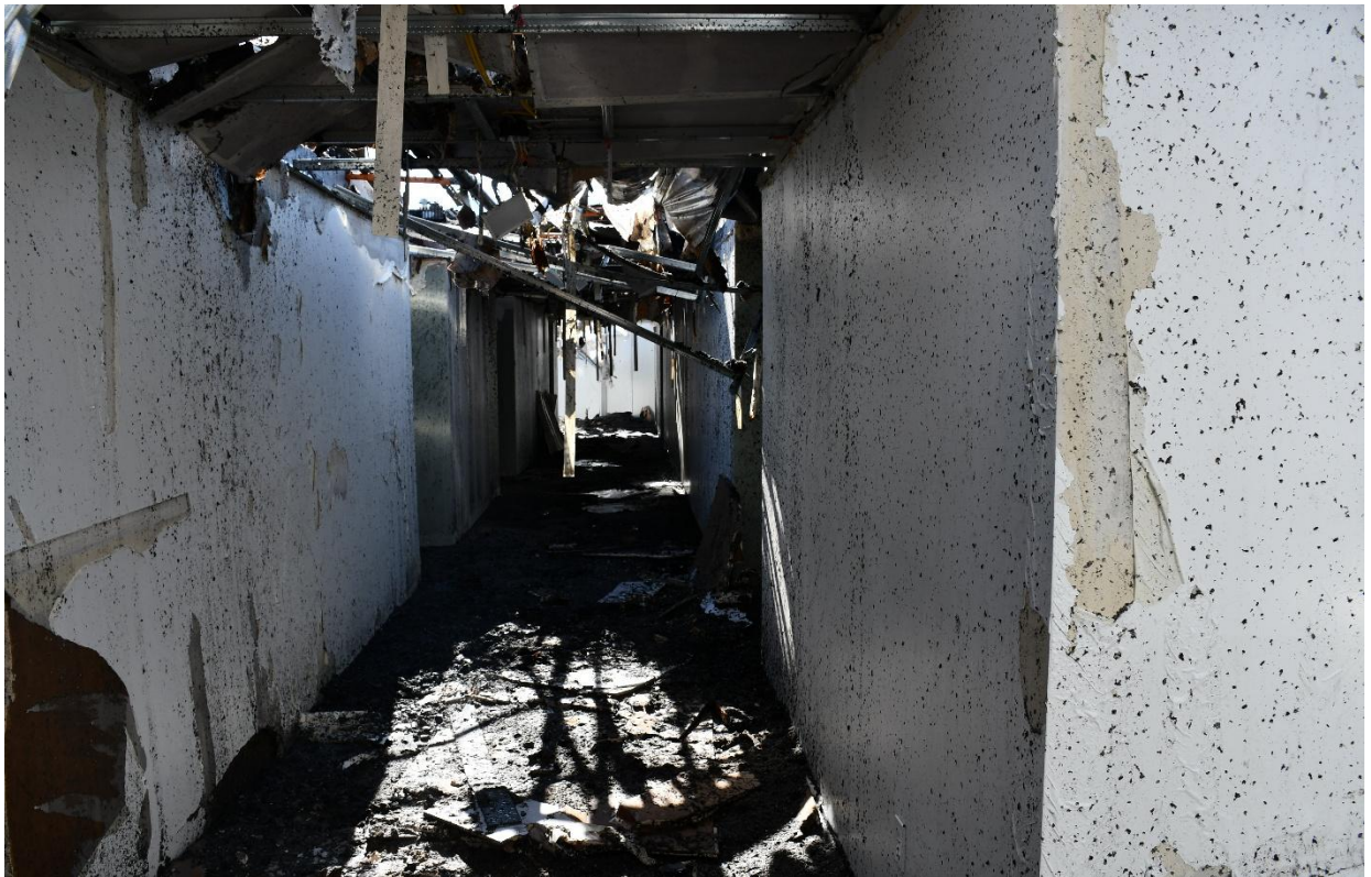
Figure #47 Looking down Hallway on 4 th floor
