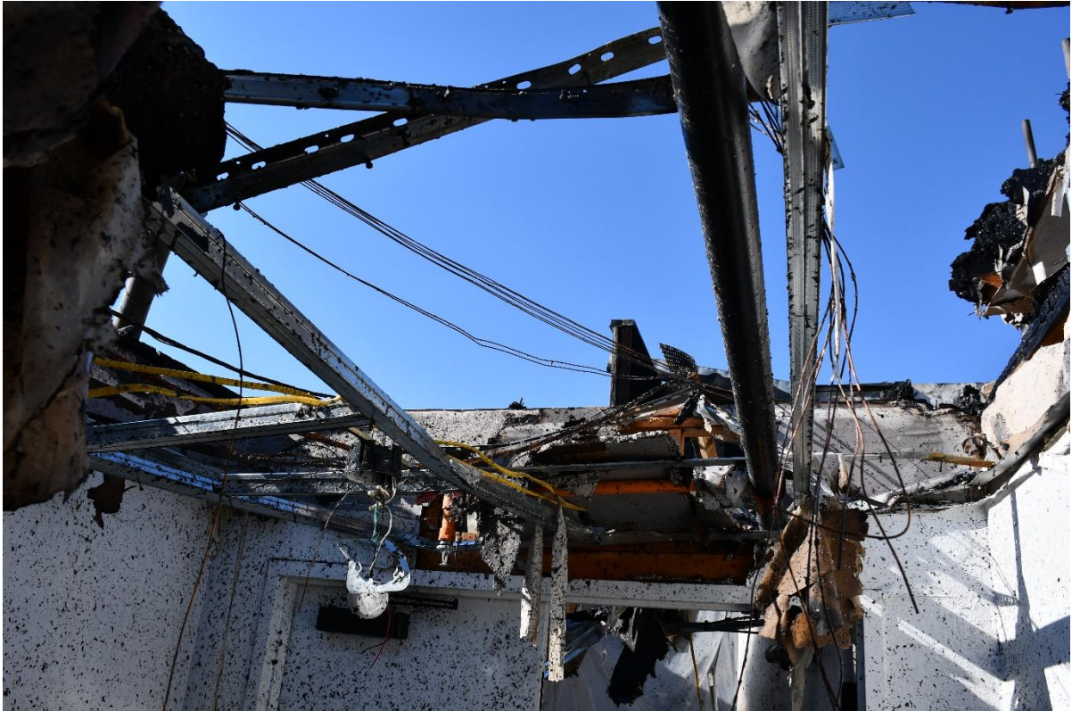
Figure #44 Looking up from floor level
