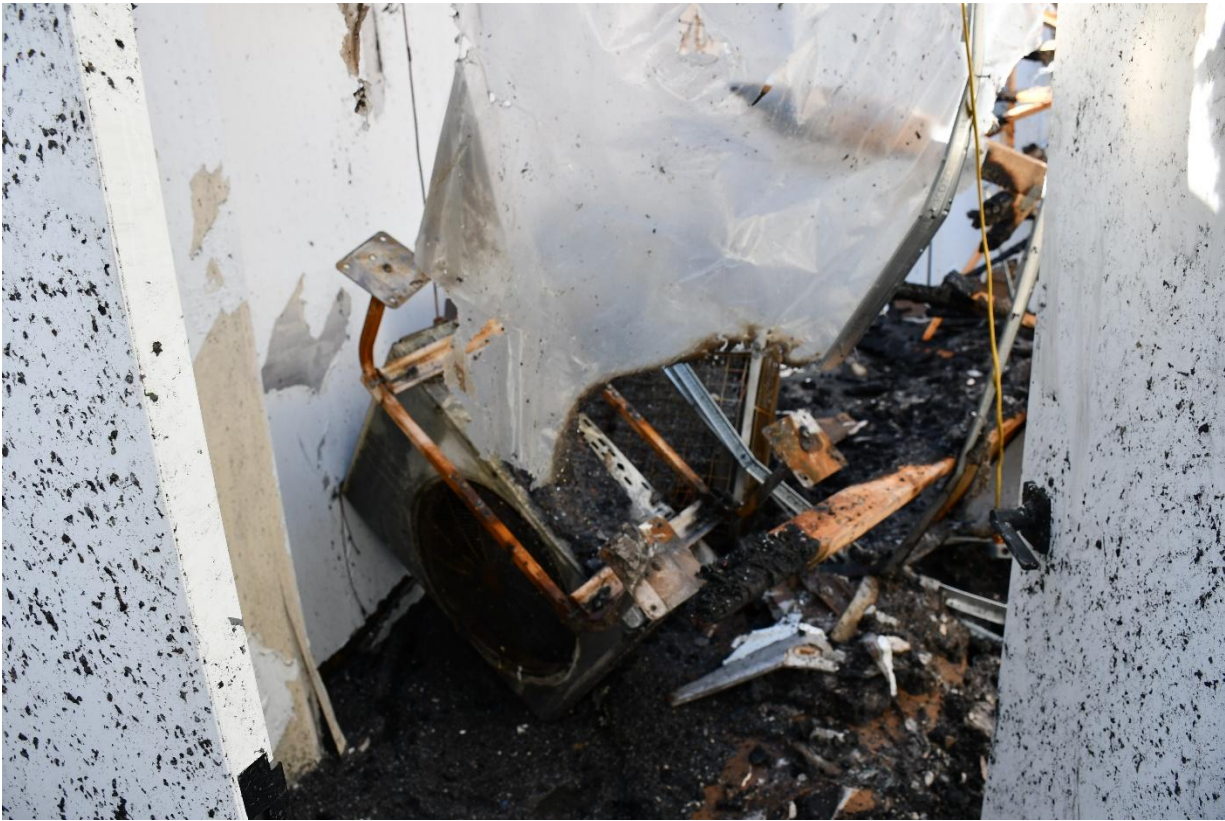
Figure #49 air-conditioning units & Debris in collapse zone
