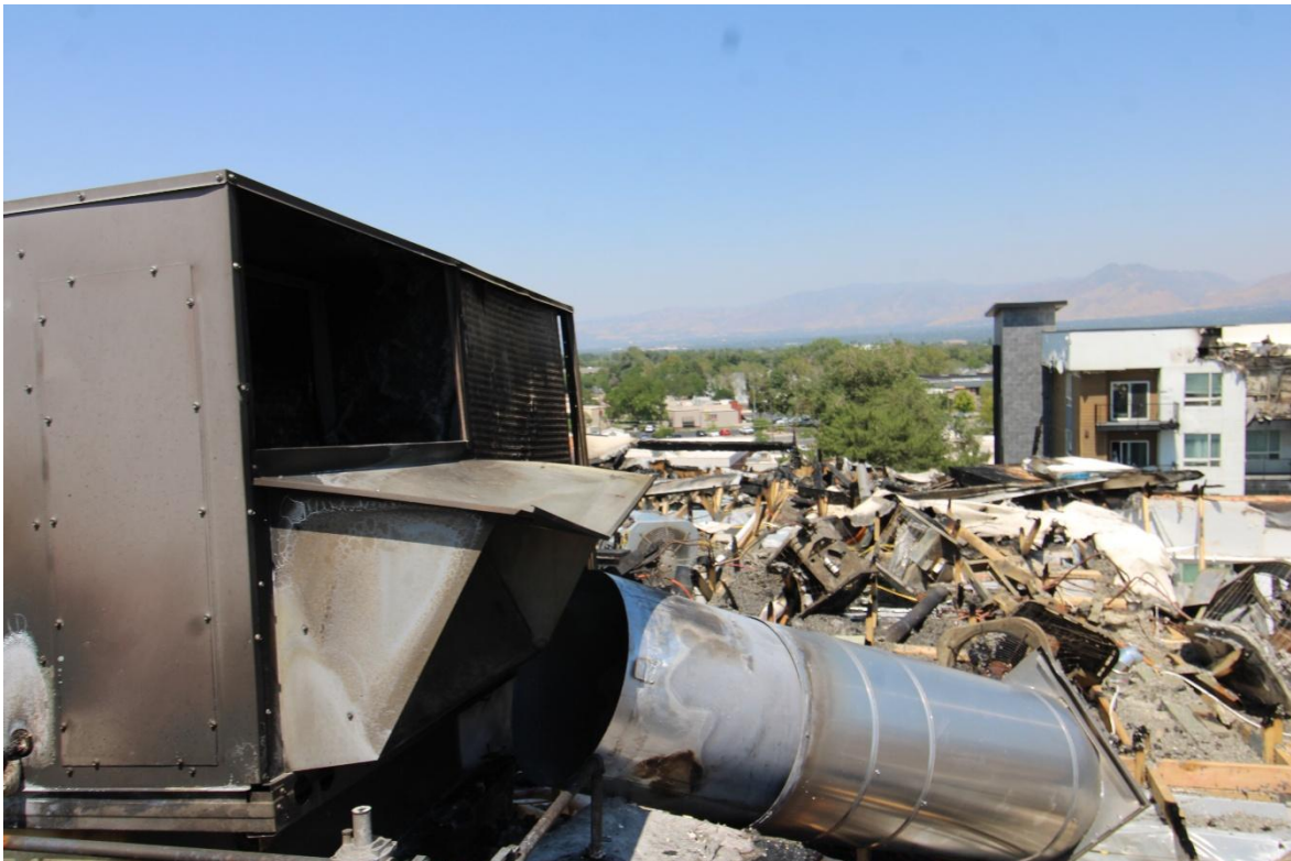
Figure #41 Looking North from Hallway opening
