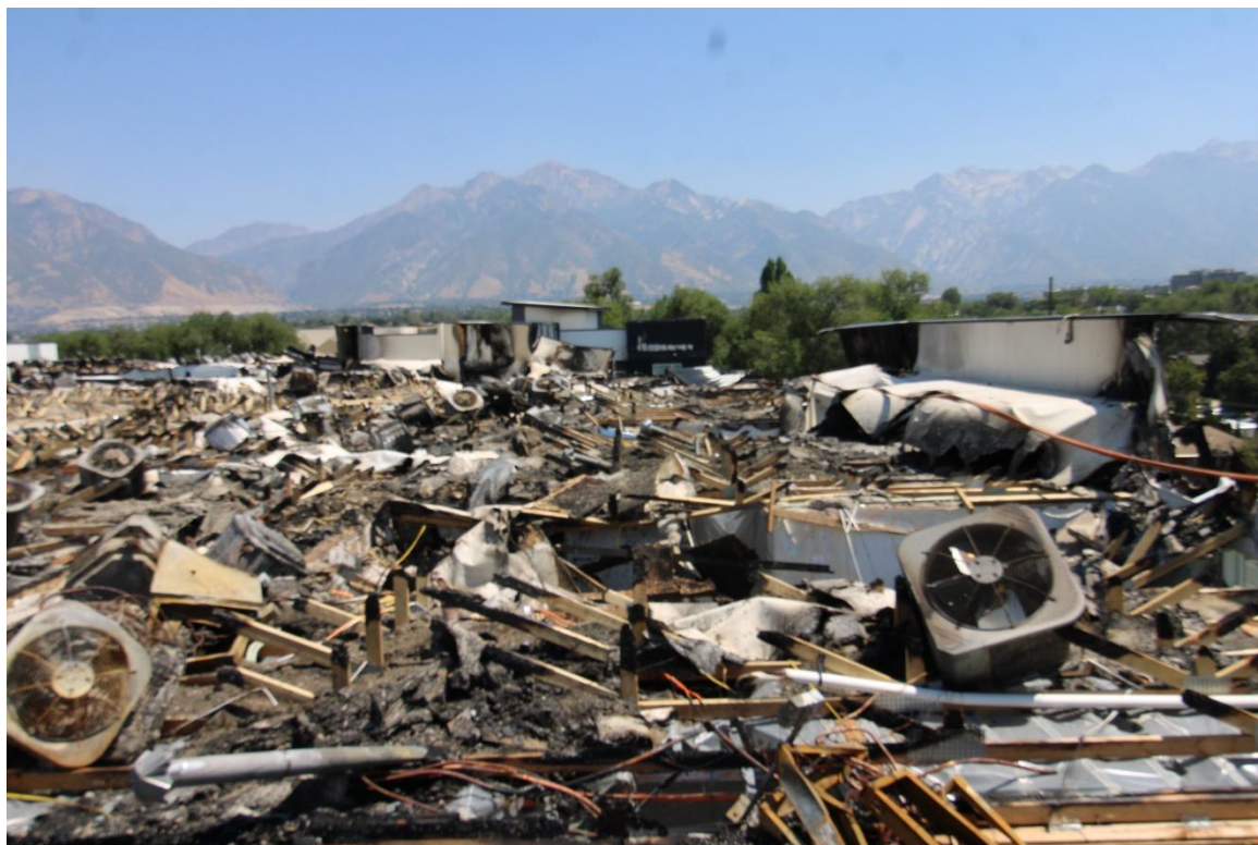
Figure #40 Looking Northeast from Hallway opening
