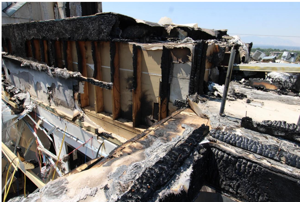
Figure #38 Close up of Elevator area
