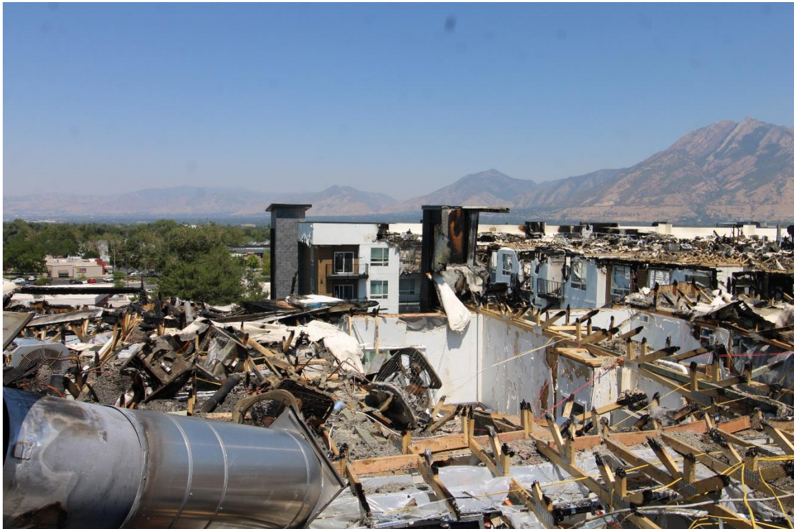
Figure #42 Looking north From Hallway opening
