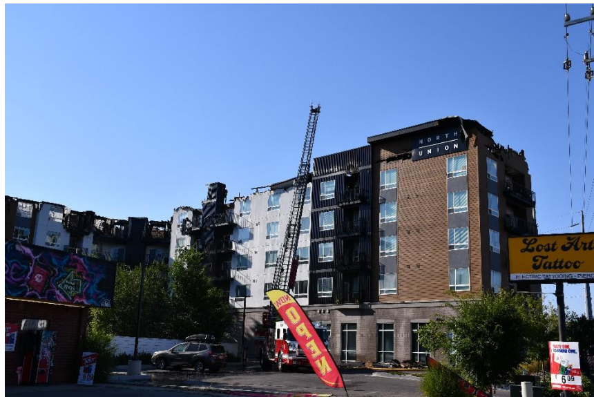
Figure #9 Looking South form parking lot by loading dock / Utility rooms
