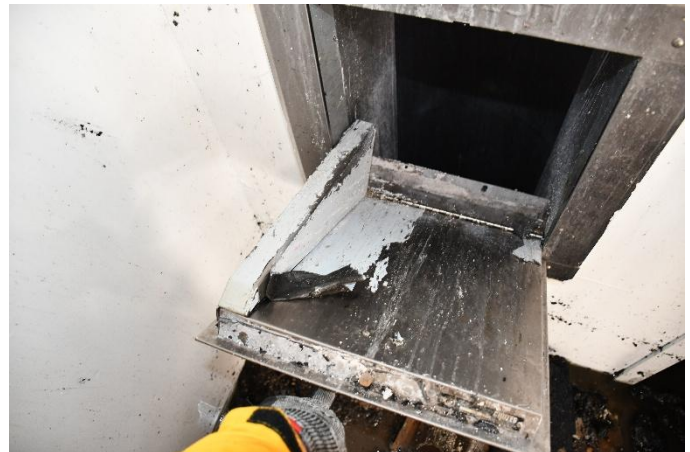
Figure 24 4 th floor Opening the garbage shoot
