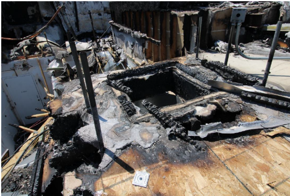
Figure #36 another angle from Hallway towards the elevator
