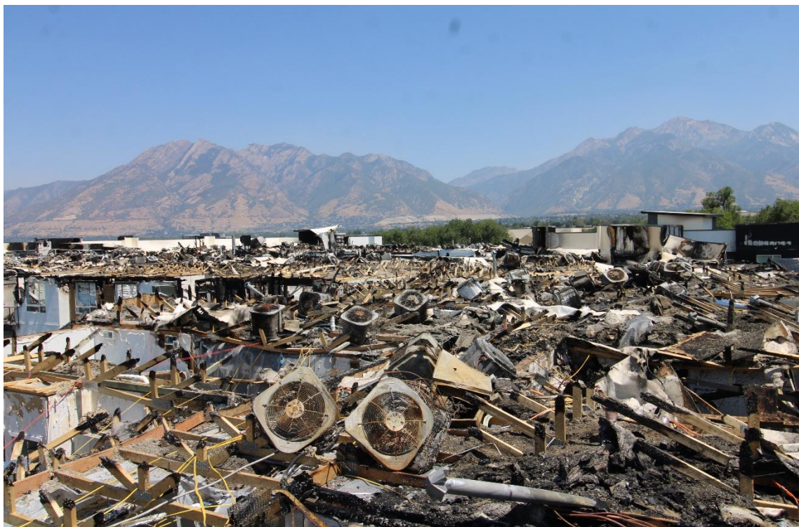
Figure #39 Looking East from hallway opening
