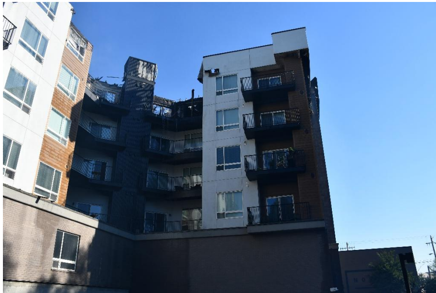
Figure #13 Looking at the upper section of Northeast side of building
