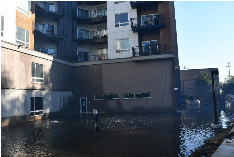
Figure #12 Looking at the lower section of the East side of the building
