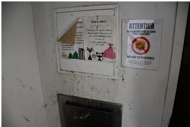
Figure 23 4 th floor outer wall of garbage shoot
