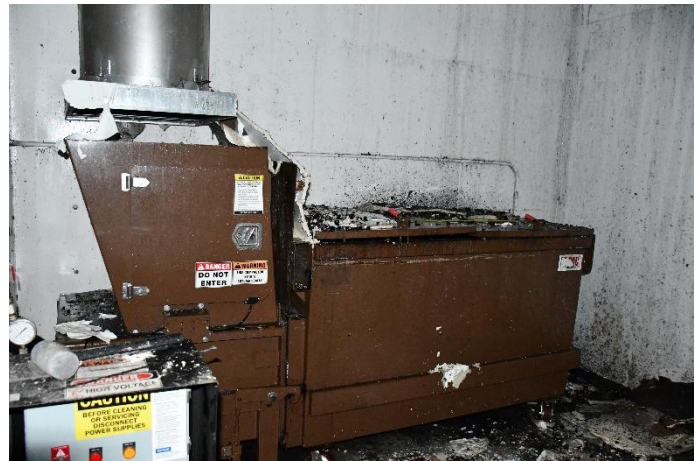
Figure 27 garbage collector/ compactor
