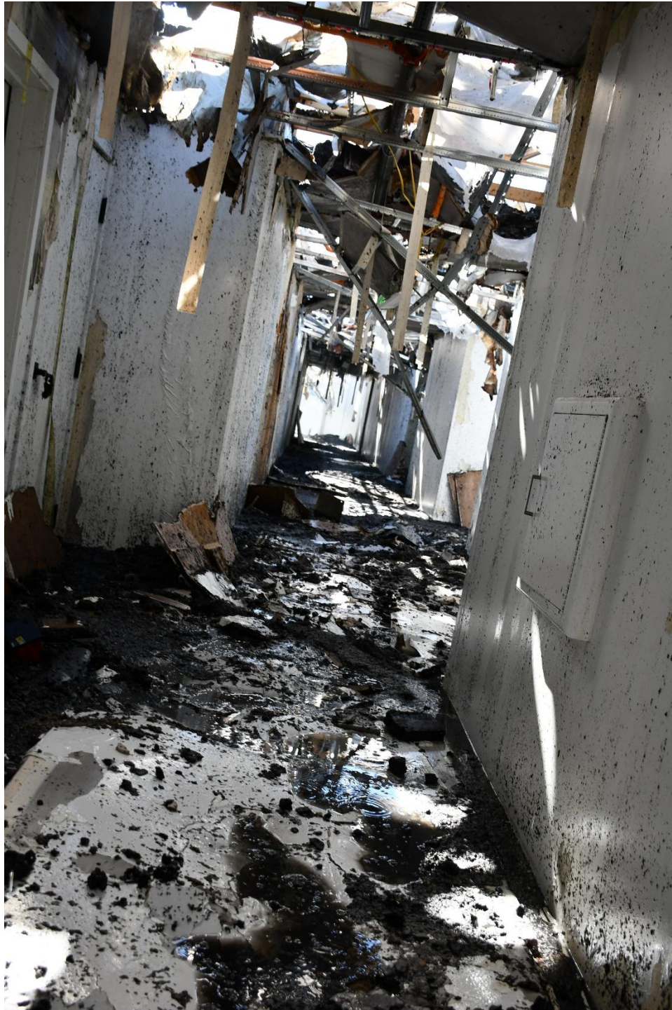
Figure #48 Looking down Hallway on 4 th floor
