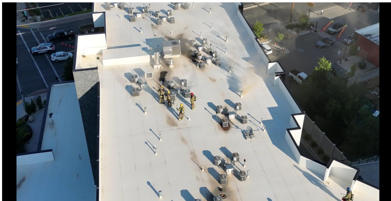
Figure #17 Rooftop screen shot from Drone video of area of origin
