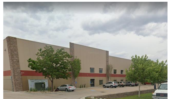
Image 28 - UFA Logistics and UTTF1 Warehouse
