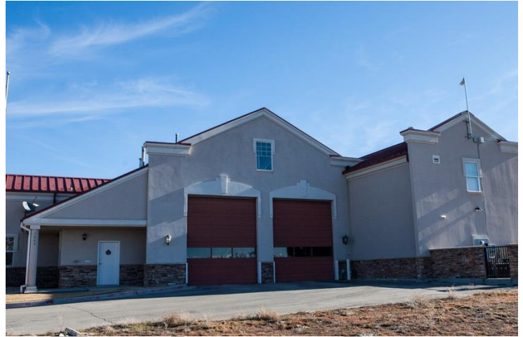
Image 9 – Eagle Mountain Station 251
