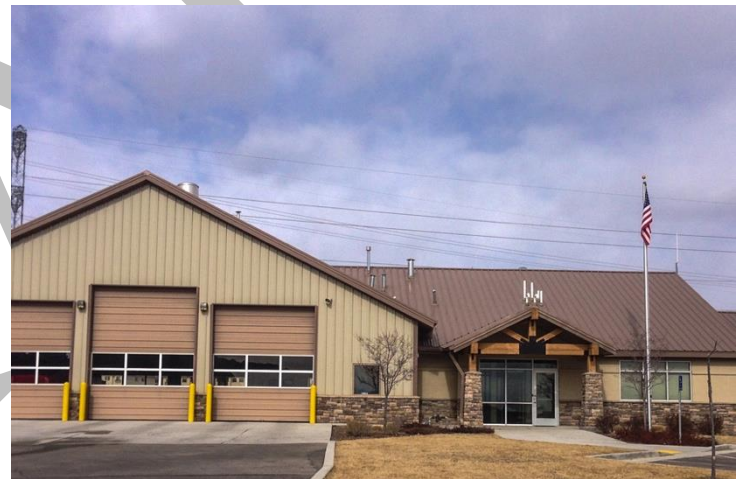
Image 10 – Eagle Mountain Station 252
