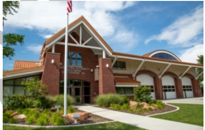
Image 21 – Millcreek City Station 106
