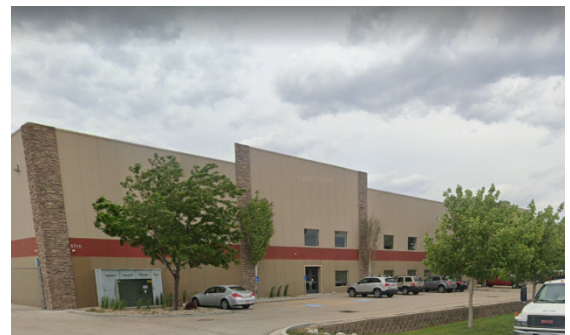
Image 28 - UFA Logistics and UTTF1 Warehouse
